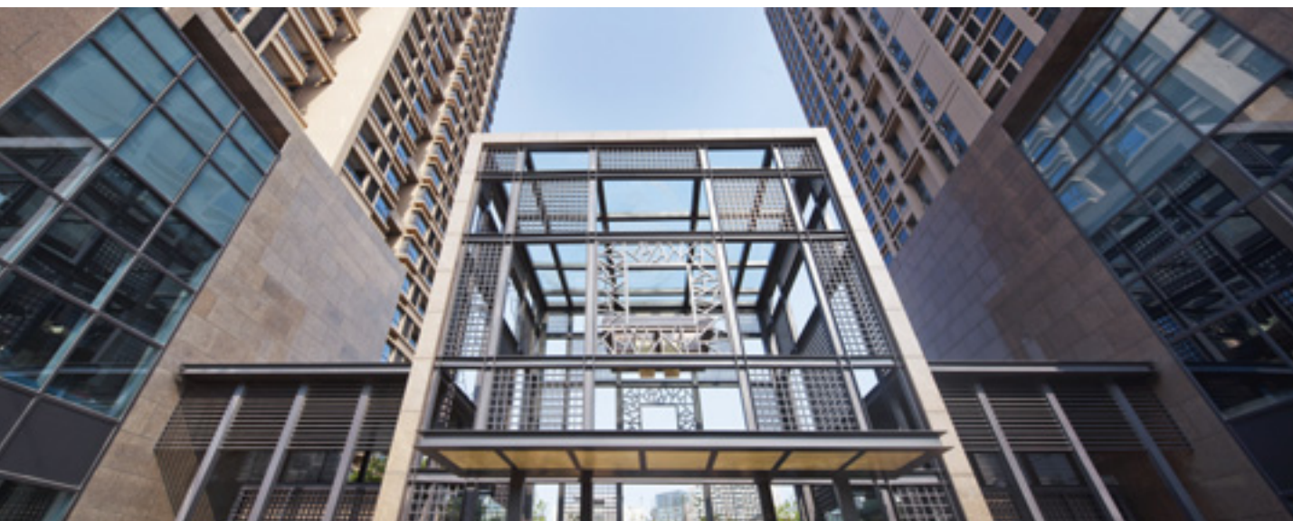
Rui Hong Xin Cheng is the first sustainable development community in East China that achieved the LEED – Neighborhood Development Pilot Version Stage 2 Gold level (Pre-certification)
