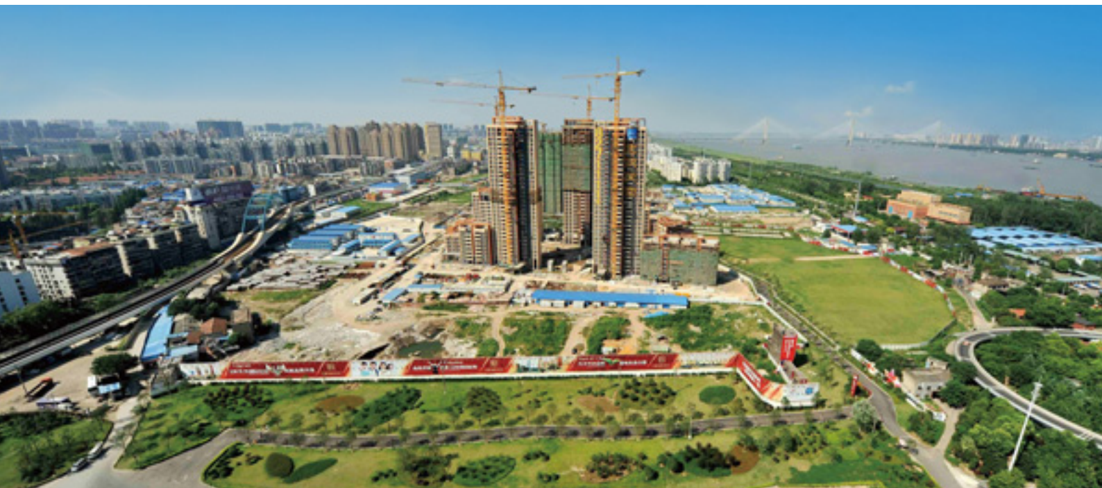
Construction site of Wuhan Tiandi
