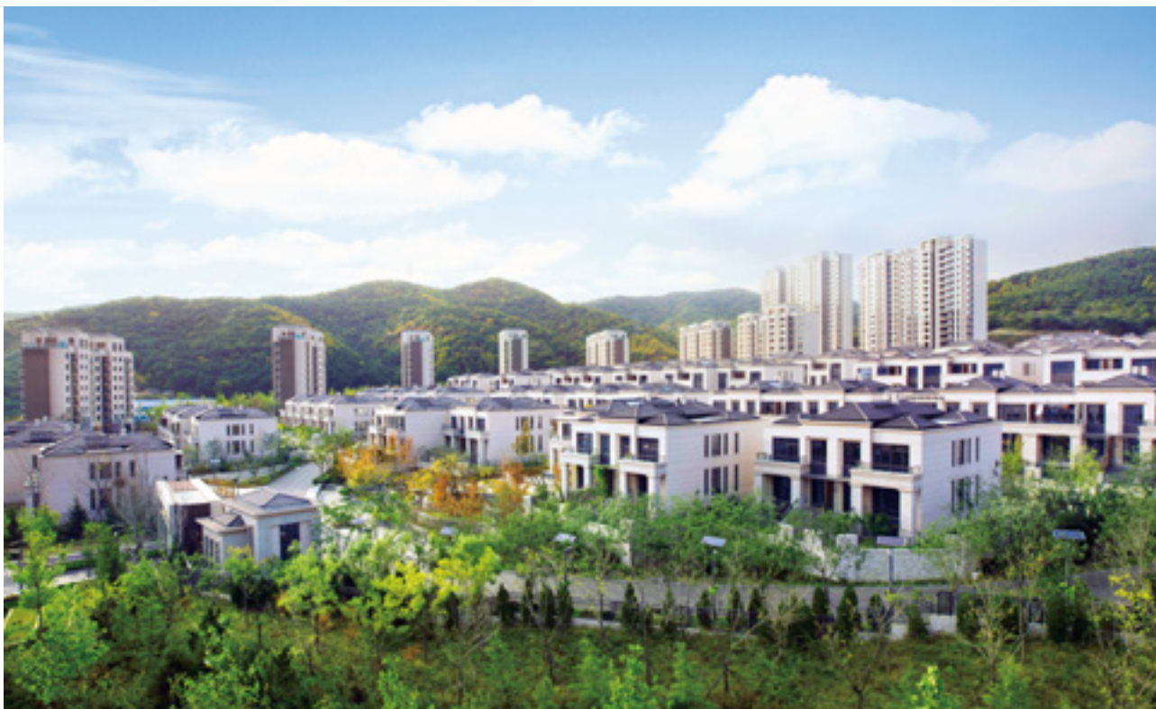
Greenville at Dalian Tiandi
