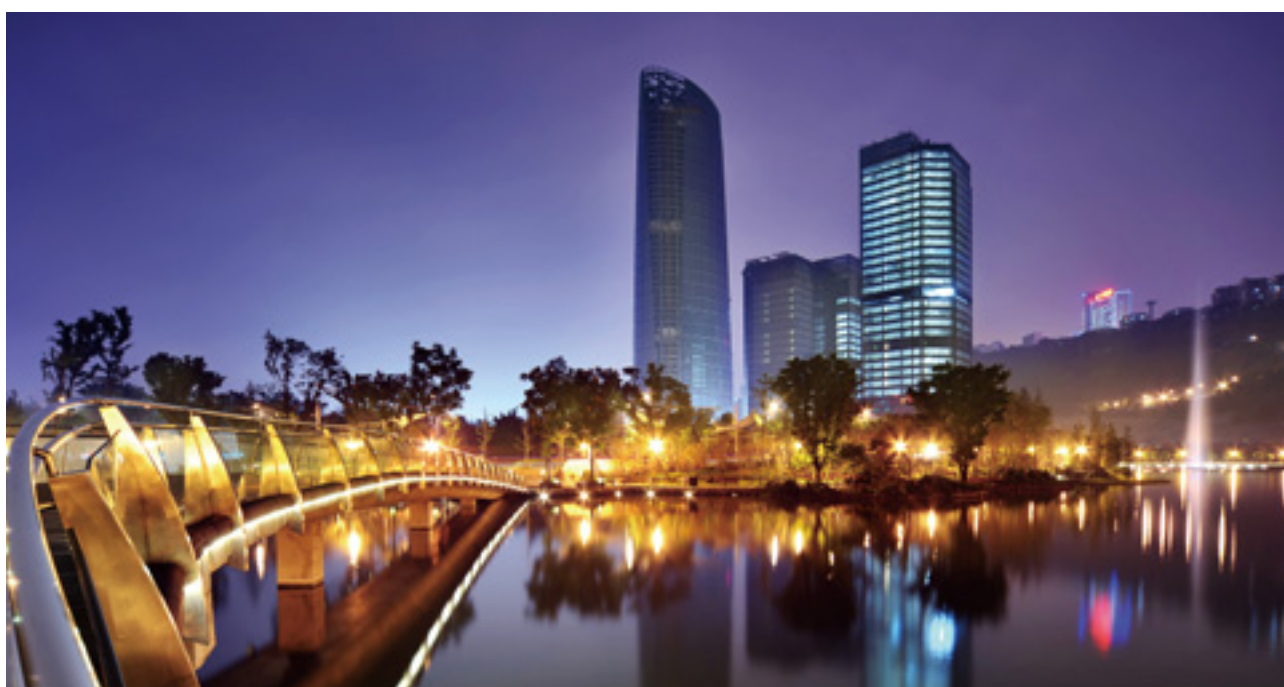
Lakeside view of Corporate Avenue at Chongqing Tiandi
