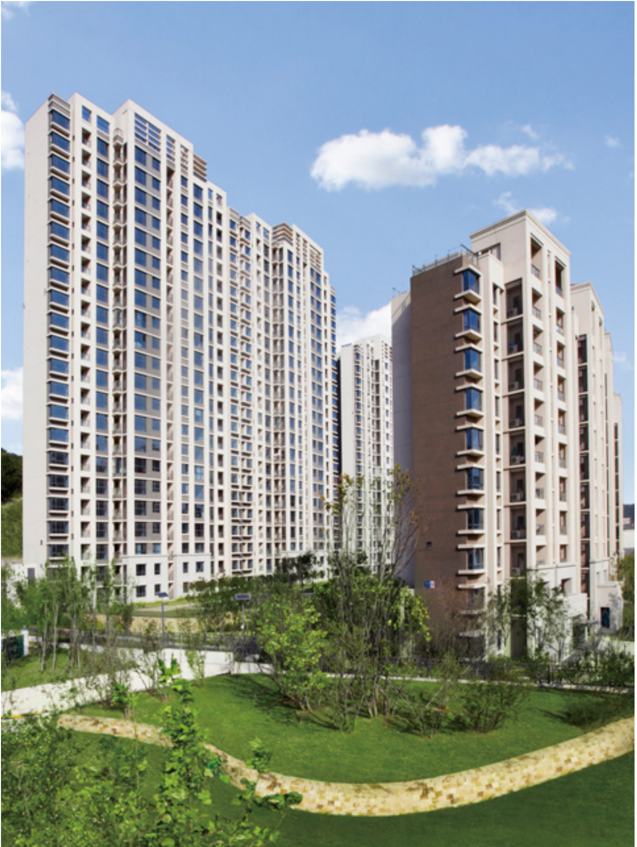
Greenville at Dalian Tiandi
