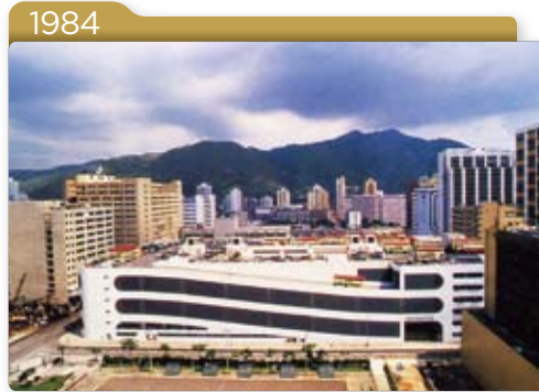
KMB's Overhaul Centre, listed in the Guinness Book of World Records as the largest multi-storey bus depot in the world, became operational
