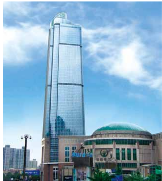
Office Tower II, The Grand Gateway, Xuhui District, Shanghai
