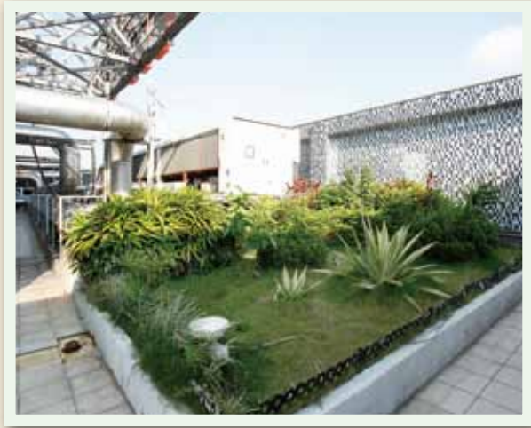
▲ Green roof at AIA Tower
