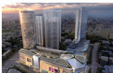
鄭州悅府 Zhengzhou MIXc Residence
