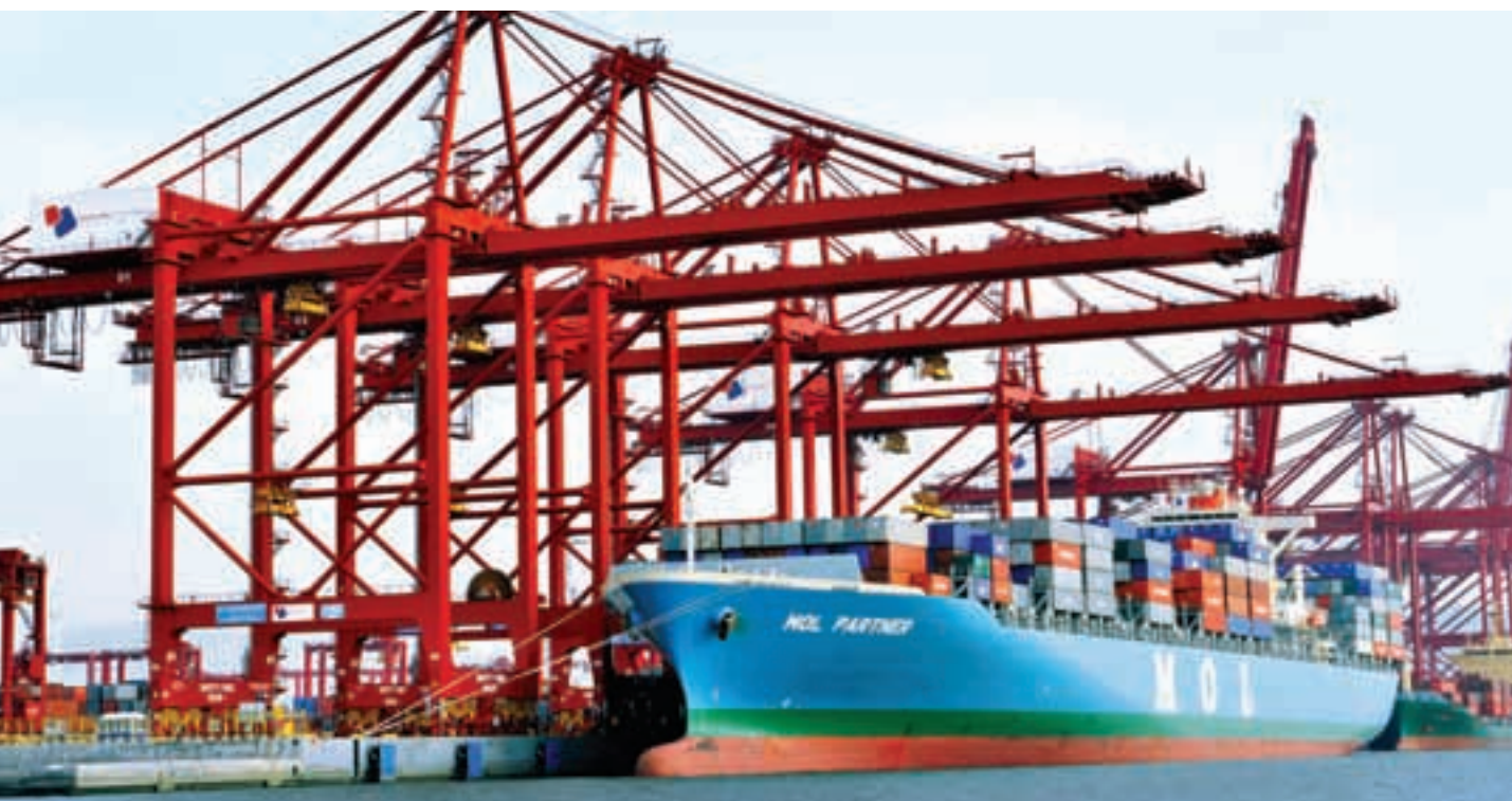
Da Chan Bay Terminal One in Shenzhen
