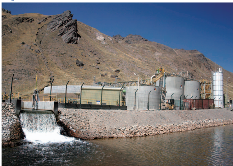
Kingsmill Tunnel Water Treatment Plant 金新米爾隧道污水處理廠
