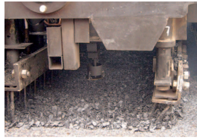
Rake the softened pavement and apply rejuvenating agent to aged asphalt
