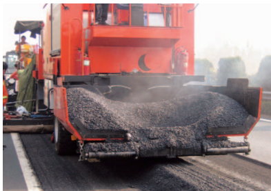
Add new asphalt mixture onto original asphalt mixture to create a recycled mixture
