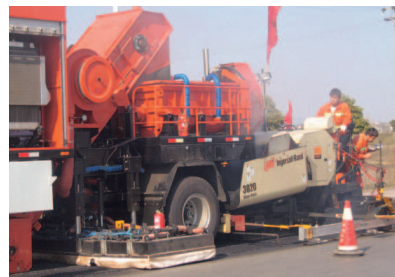
Fully blend the recycled mixture and reheat the pavement surface using thermal bonding technique
