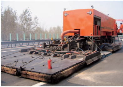
Heat and soften the original pavement
