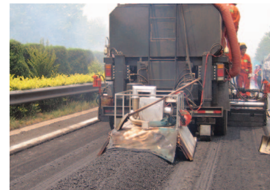
Collect the original asphalt mixture into a single row
