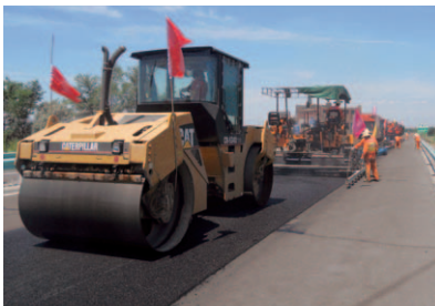
Compact the new pavement
