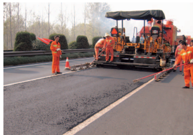
Pave the fully blended recycled mixture
