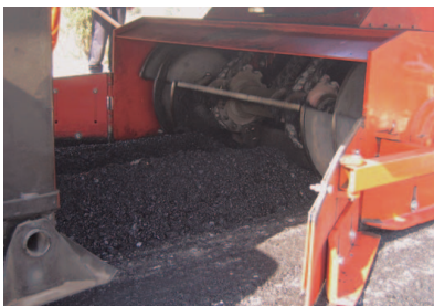
Collect and convey the recycled mixture into a mixer
