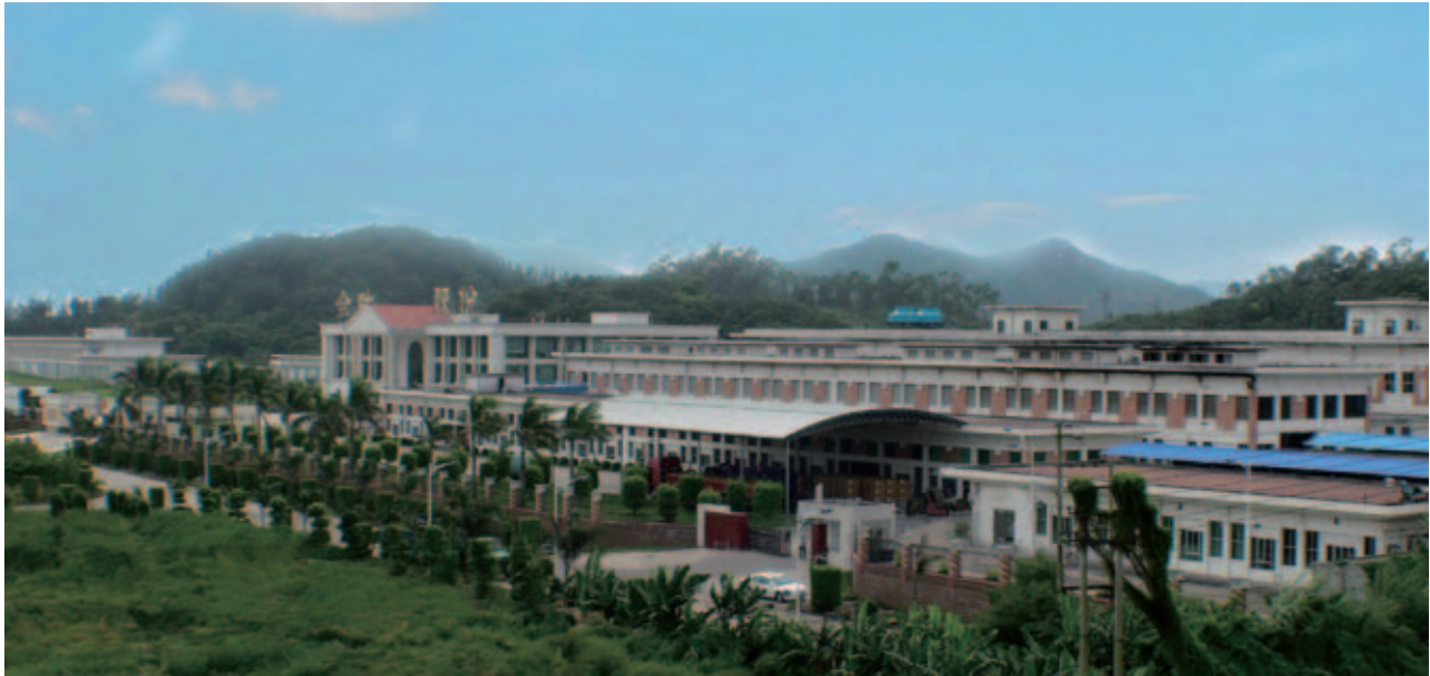
Outlook appearance of Guangdong Jinye production base and office tower in Shantou 位於汕頭的廣東金葉生產基地及辦公大樓外貌
