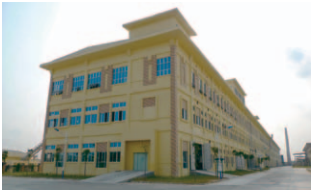
Outlook appearance of second phase of Guangdong Jinye 廣東金葉二期廠房外貌
