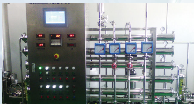
Equipment Name: Partial Equipment for Purified Water System Description: Purified Water Secondary Filtration
