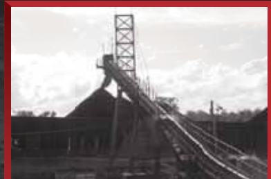
Barge Loading at Telang Baru Jetty
