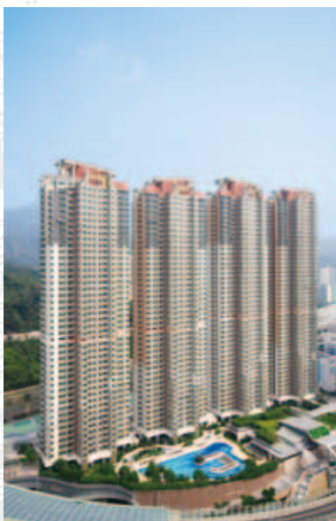
Residential development of Phase 2, Festival City at Tai Wai, Hong Kong includes four blocks. 盛薈包括4座住宅大廈，為香港大圍名城第二期住宅物業發展項目。
