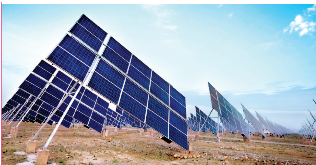
Jinchang Solar Farm – CLP's first solar project in the Chinese mainland
