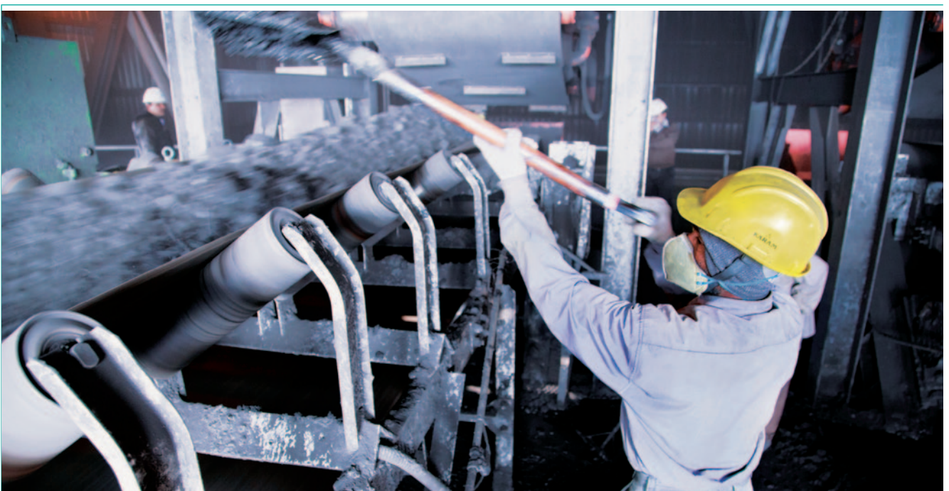
Technician performing maintenance work at Jhajjar's coal conveyor system
