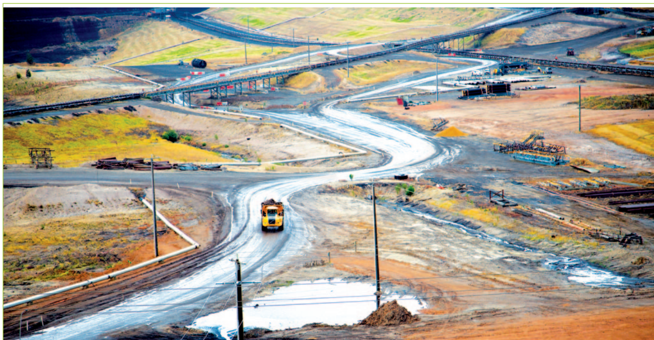
Remediation work at Yallourn
