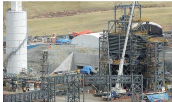
Pebbles Crushing & Reclaim Tunnel
