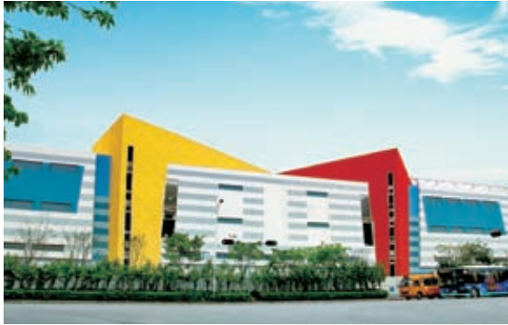
New Logistic Centre at South China Logistic Park
