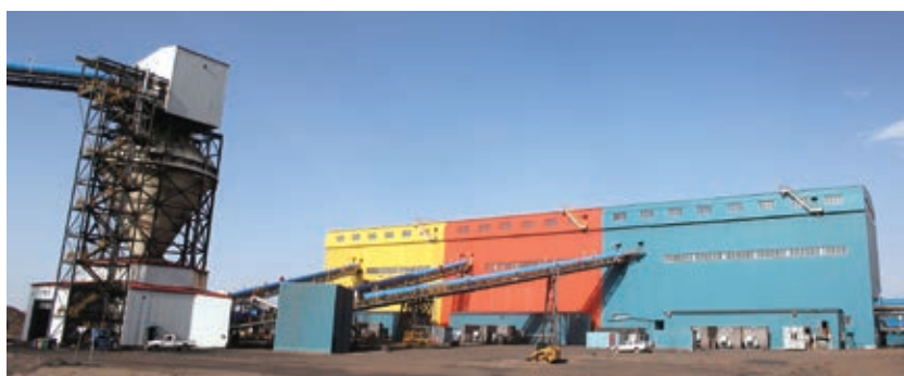
CHPP with 3 modules completed
