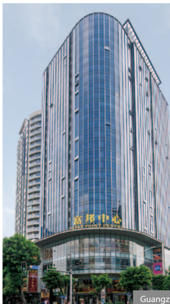
Guangzhou West Point
