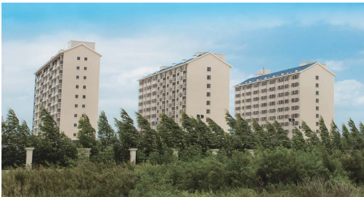
The new staff residential quarters in Quanzhou base.
