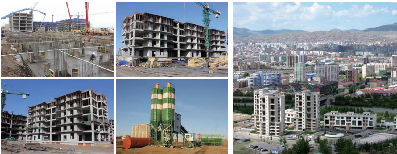
Erin Town in construction
