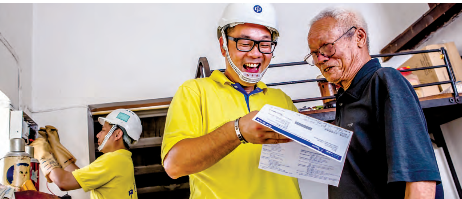
⚙️ CLP Volunteers provide rewiring service for the elderly living alone
