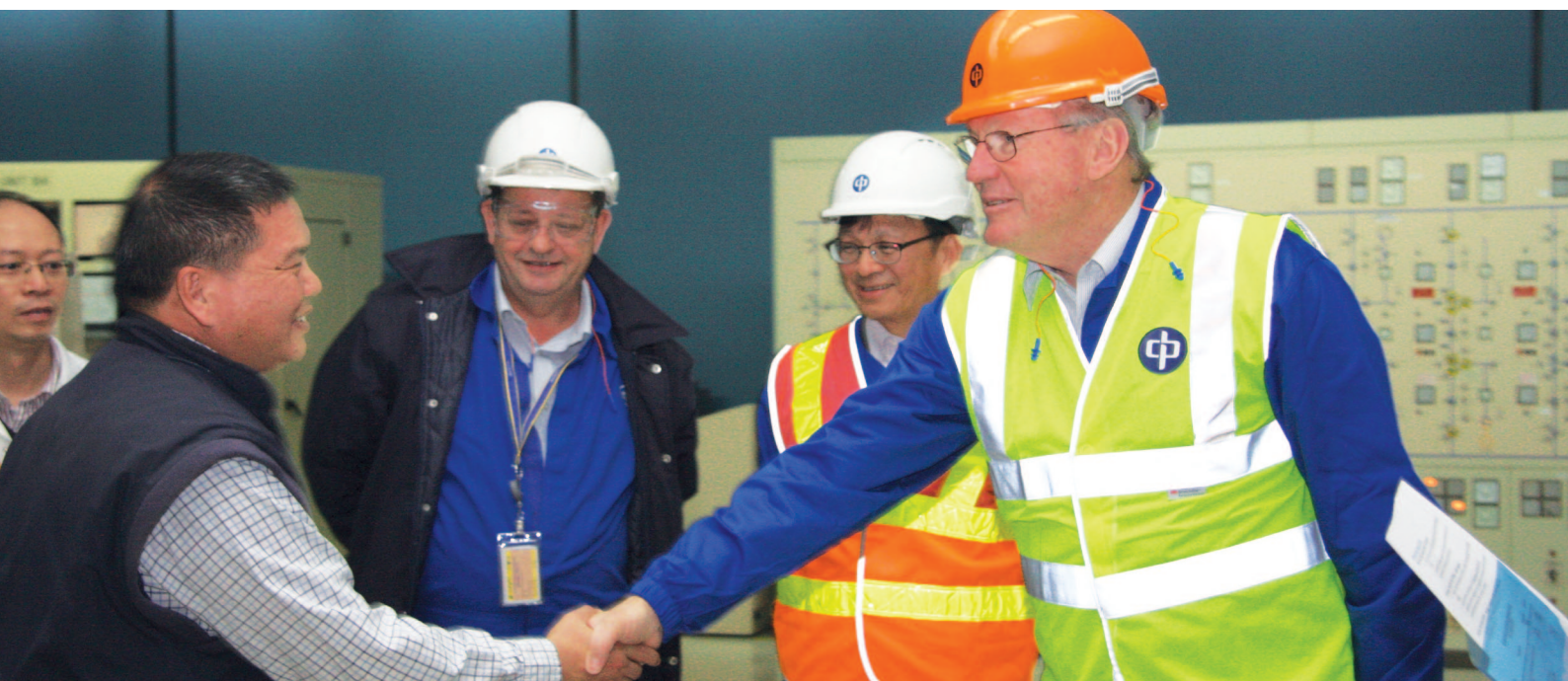
⚙ Sir Rod Eddington, Independent Non-executive Director, thanks staff during a visit to Castle Peak Power Station
