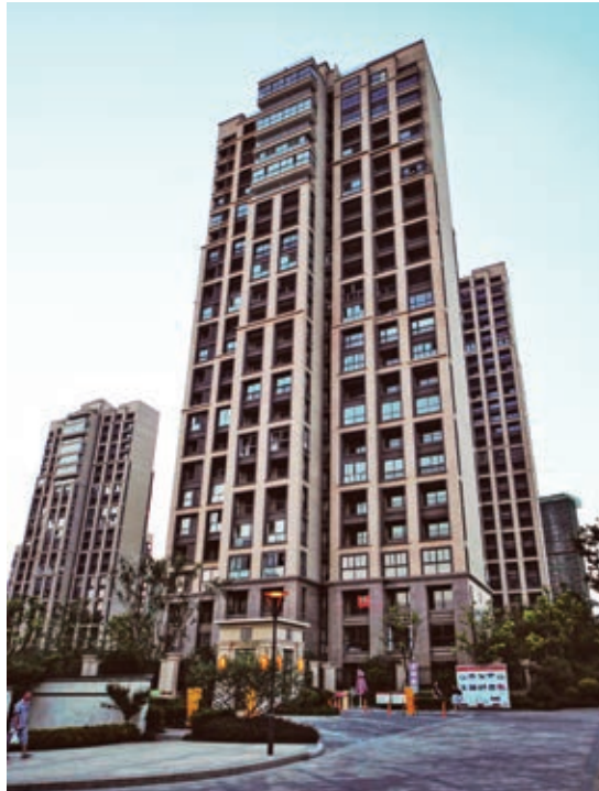
Nantong Jingrui Dignity Mansion
