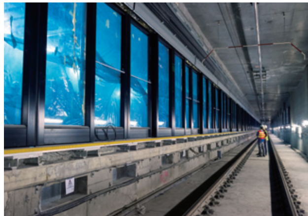
Construction of the new lines has involved extensive tunnelling work
