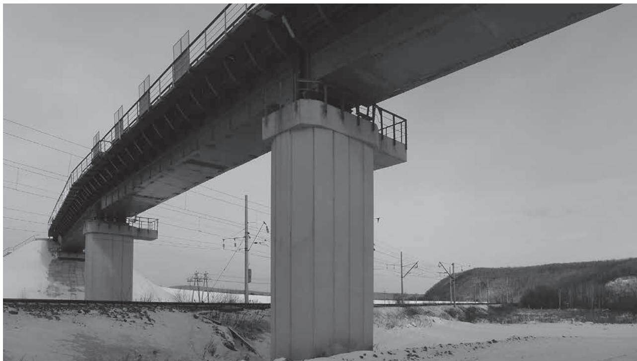
Bridge connection K&S Processing plant to Trans Siberian Railway
