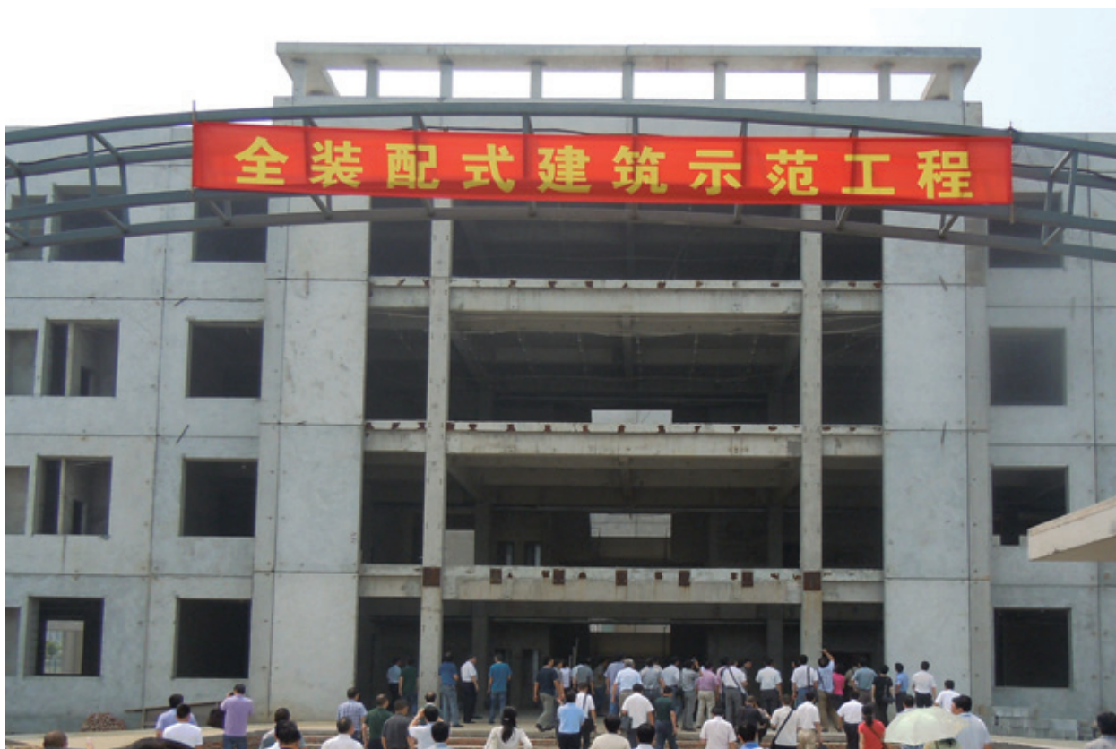
Factory of Taiyuan Environmental Protection Company (泰源環保公司), Yixing City, Jiangsu — A demonstration project of prefabricated construction in 2011
