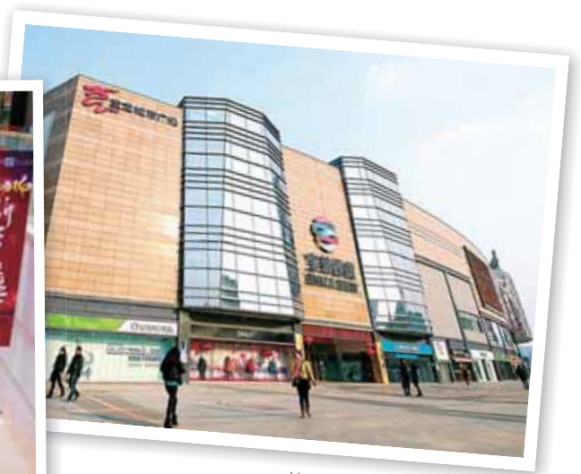
Yancheng Powerlong City Plaza
