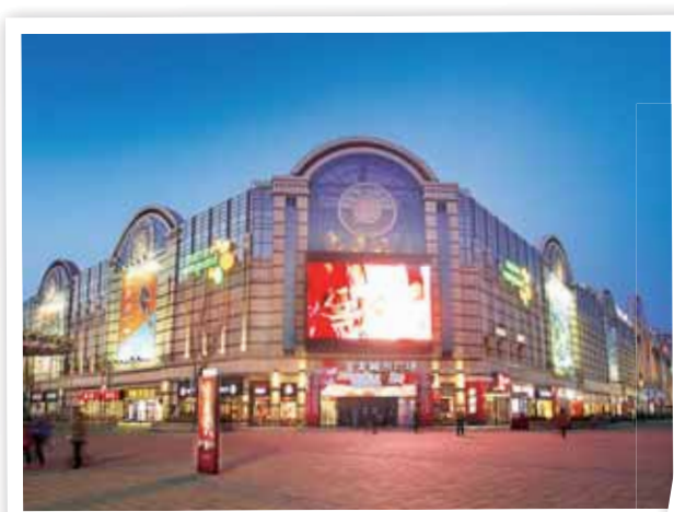
Qingdao Licang Powerlong City Plaza
