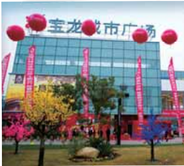
SHANGHAI CAOLU POWERLONG CITY PLAZA
