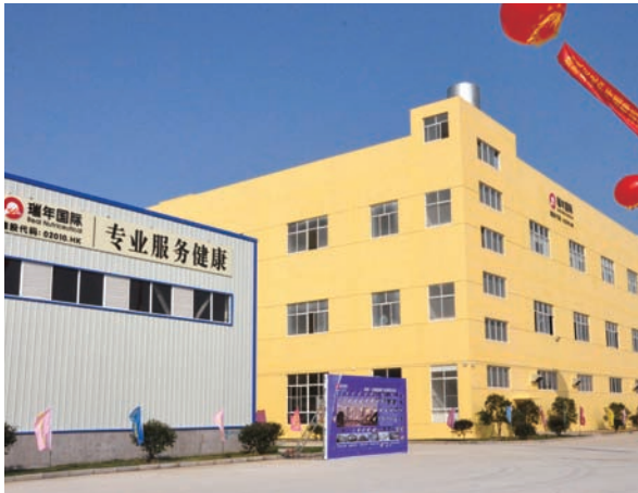
The infrastructure facilities of a new production base for health and nutritional supplements in Wuxi has been completed.
