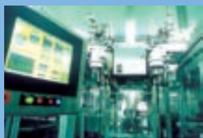
NJCTT's production plant for PVC-free large volume injections
