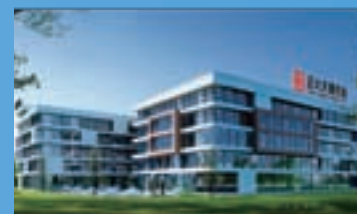
CT Tianqing's R&D Centre
