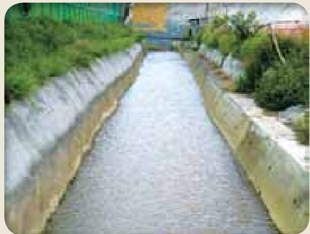
Channels to store rainwater for water-spraying at construction sites
