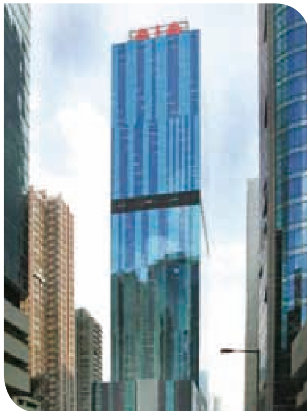
AIA Tower, North Point, Hong Kong
