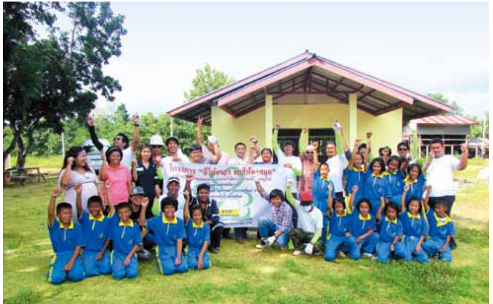
Our Volunteer Service Team in Thailand helped a local school to repaint its library and renovate its facilities.
