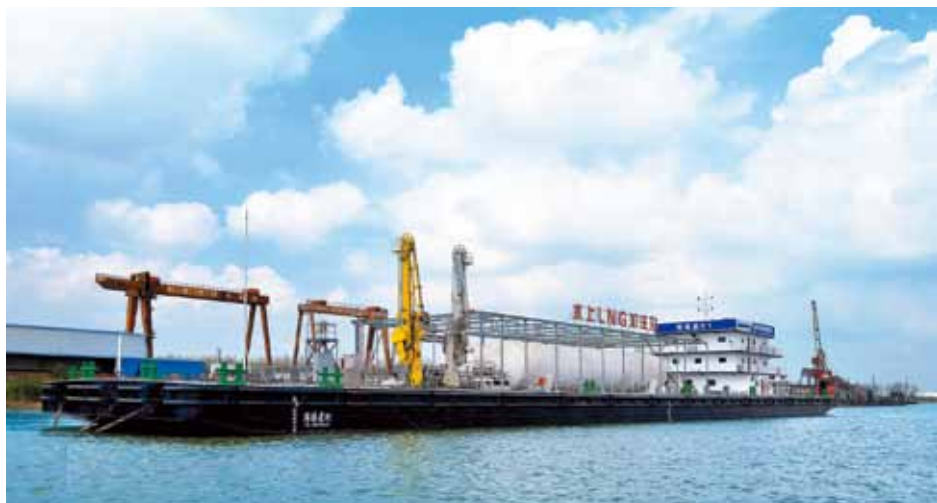
We opened China’s first inland LNG fuelling station for vessels on the Yangtze River in Nanjing, Jiangsu province.
