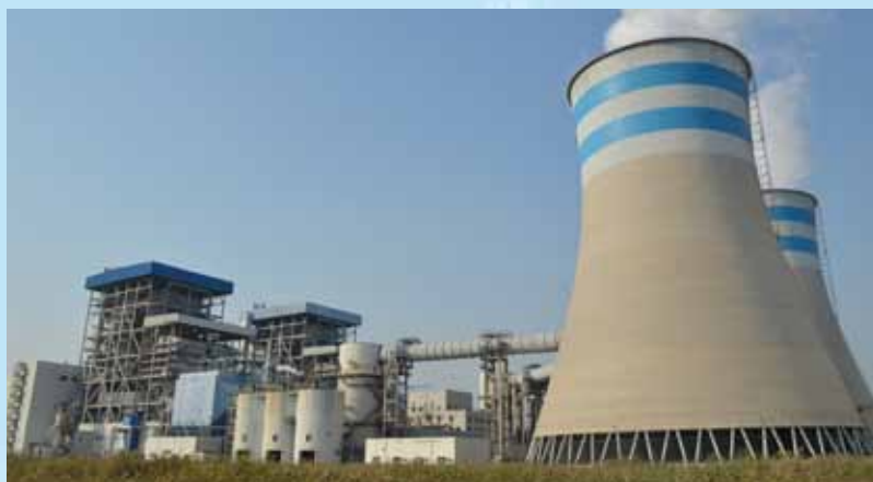
Guodian Group's first desulfurization project adopting a system of a combination of no bypass and smoke tower
