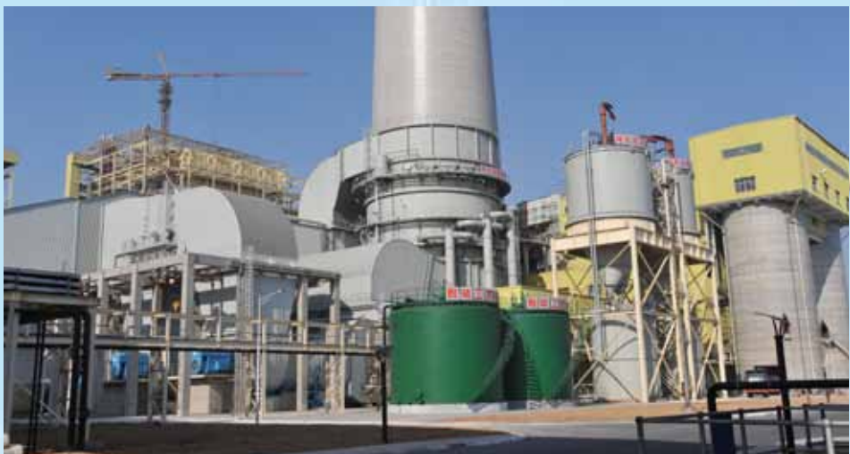
The PRC's first power generating unit with a million kW that performs desulfurization and denitration at the same time.
