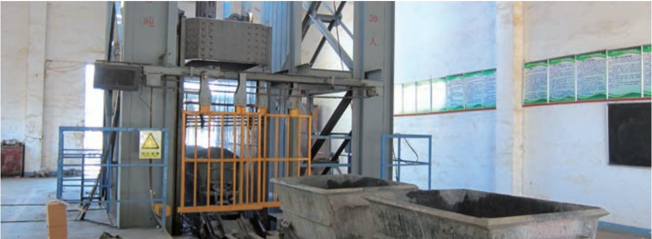
The central secondary shaft at Daxin Mine
