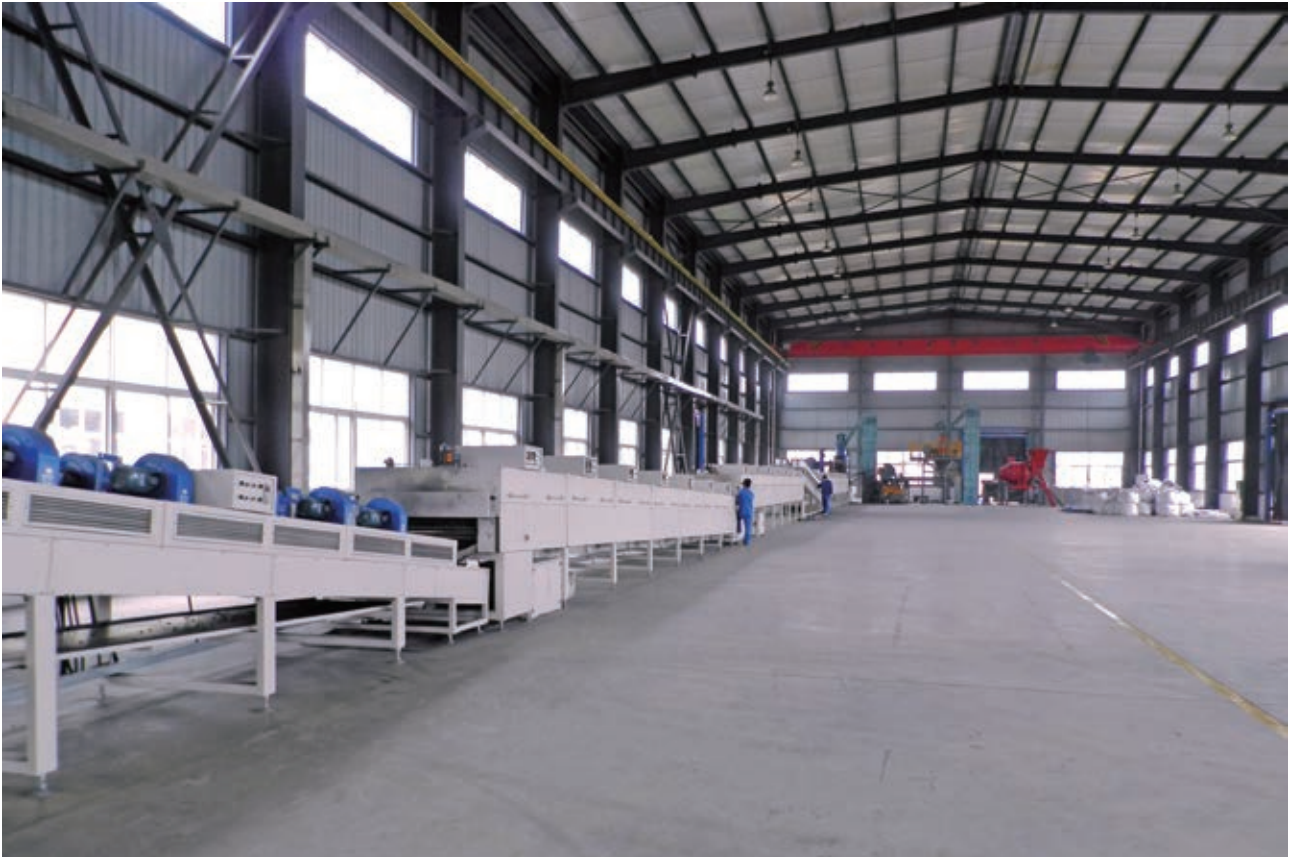
Manganese briquette production line at Chongzuo Branch
