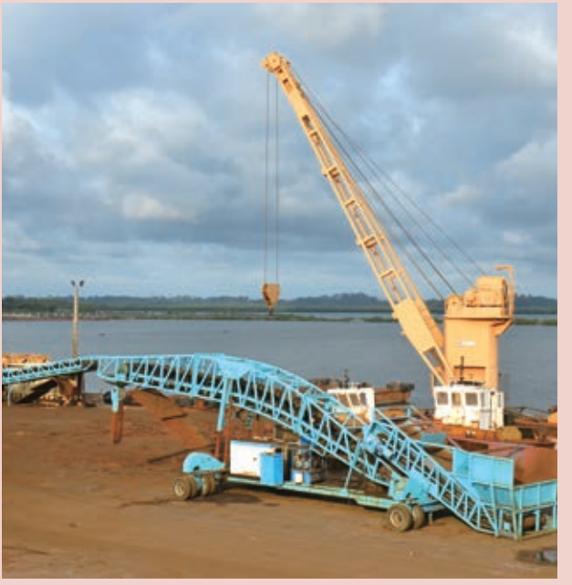
The manganese concentrates are loaded to the barge through the belt transporter
