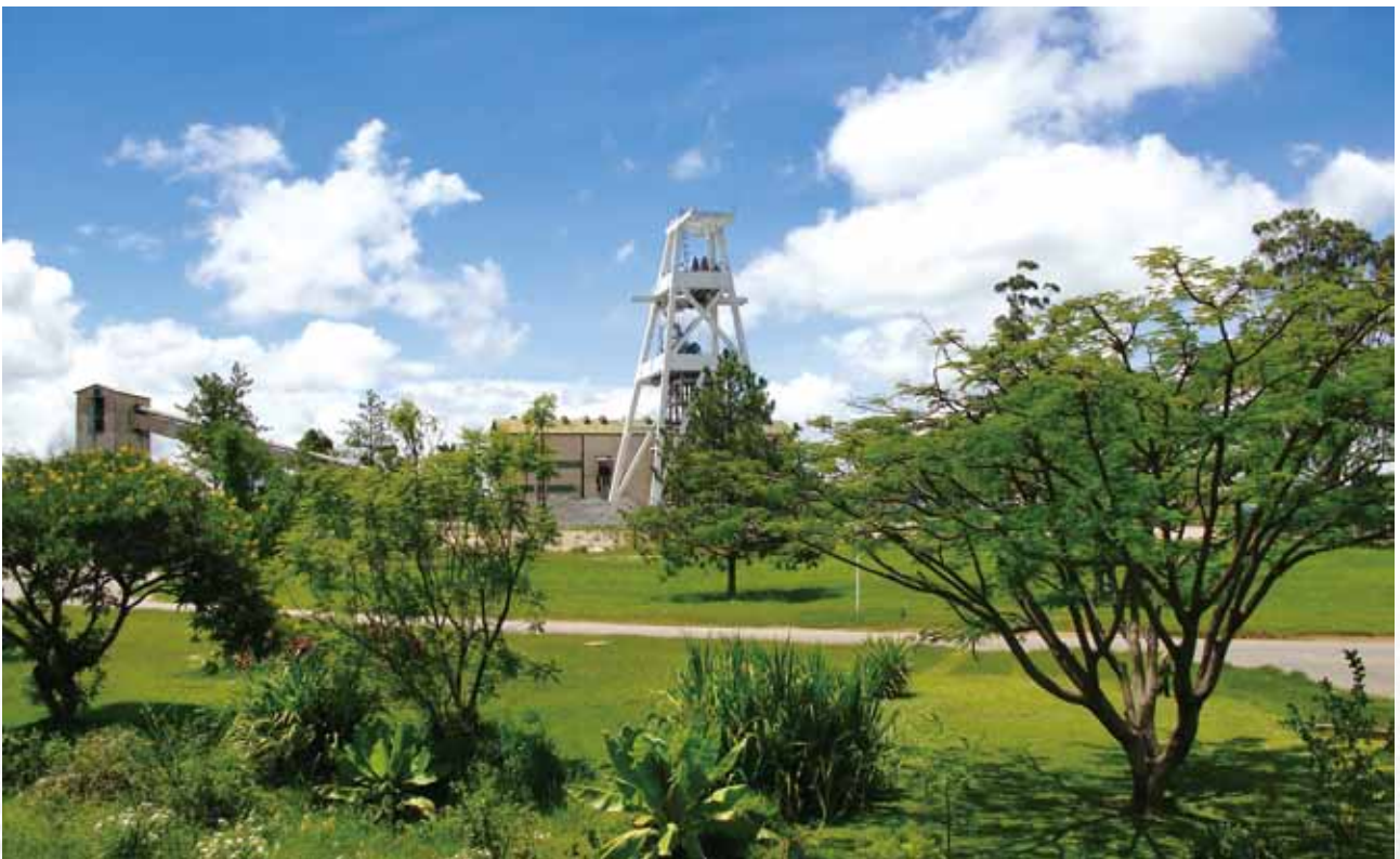
Chambishi銅礦主井架
