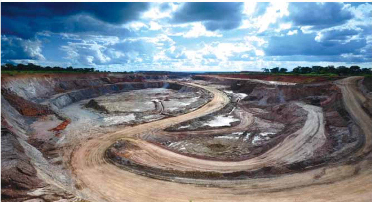
Surface mine of Muliashi Project
