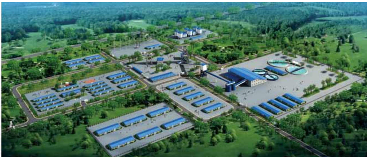
Bird's-eye view of mining and processing engineering of Chambishi Southeast Mine
