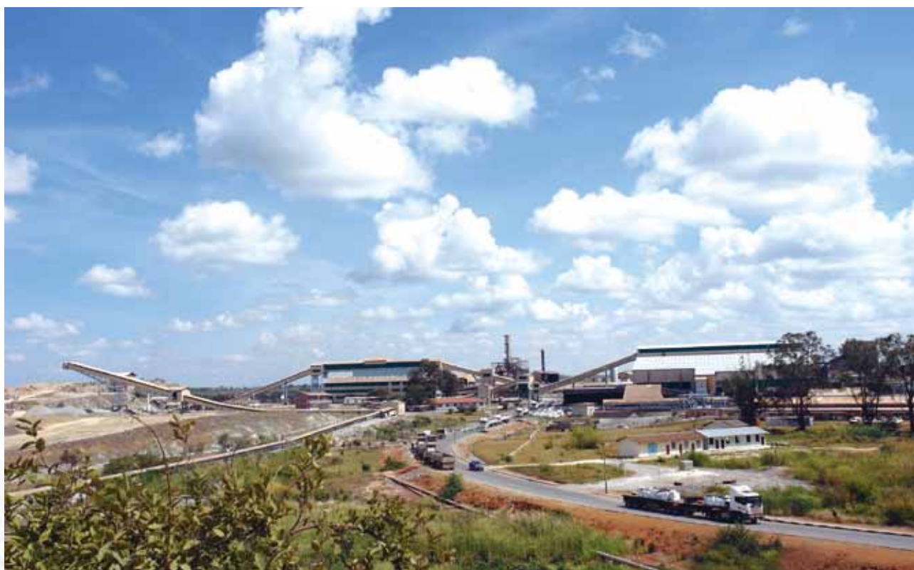
Panorama of the ore processing plant of Chambishi Copper Mine
