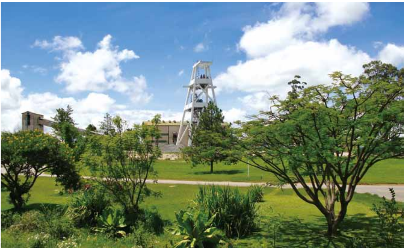
Main shaft of Chambishi Copper Mine
