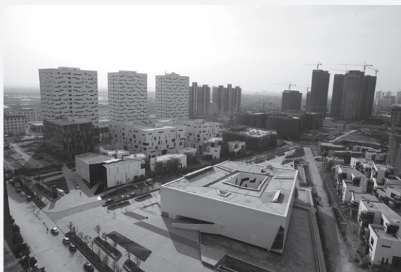
Creative Capital (Phase I) under construction
