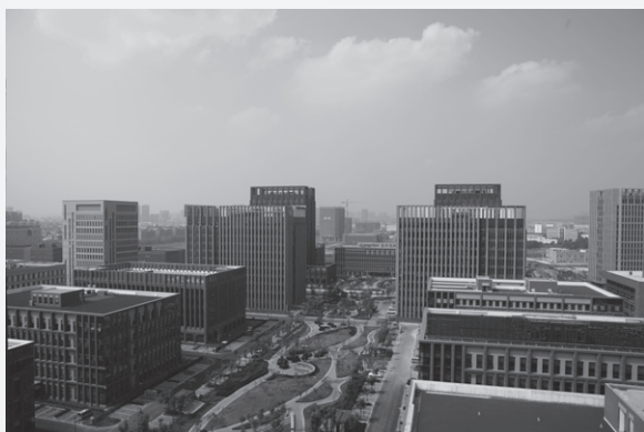
Phase II — Buildings B1–B20 completed
