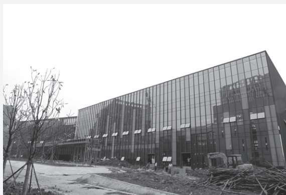
Phase II — Buildings B21–B30 under construction
