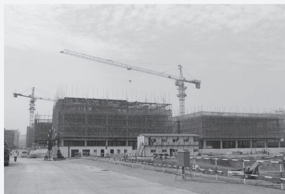
Areas 1.3 and 1.4 under construction
