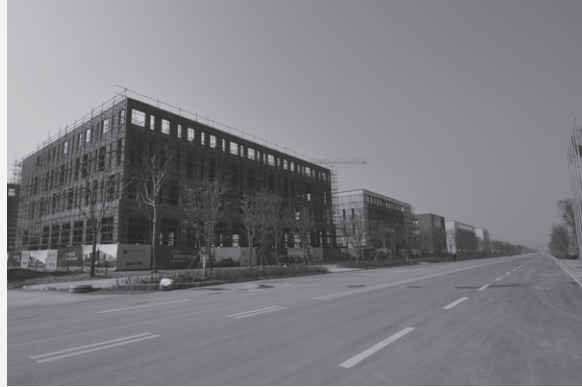
Phase I — Area 1.1 — Clusters C7-C9 under construction
