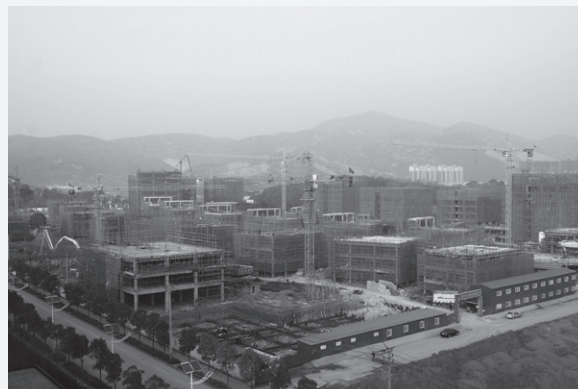
Phase I under construction
