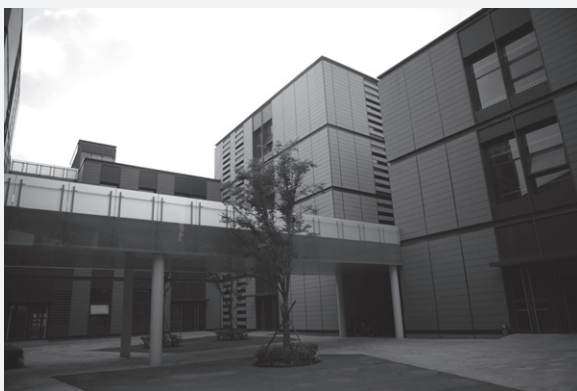
Areas 1.1 and 1.5 completed
