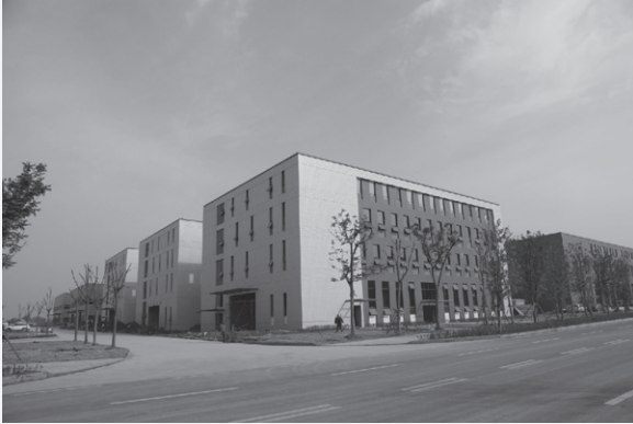
Phase I — Area 1.1 — Clusters D2-D3 and D5-D6 completed
