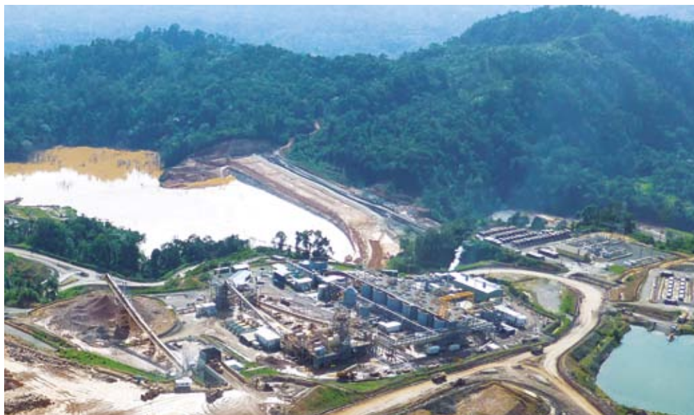
Aerial view of site facilities showing process plant and tailings storage.
