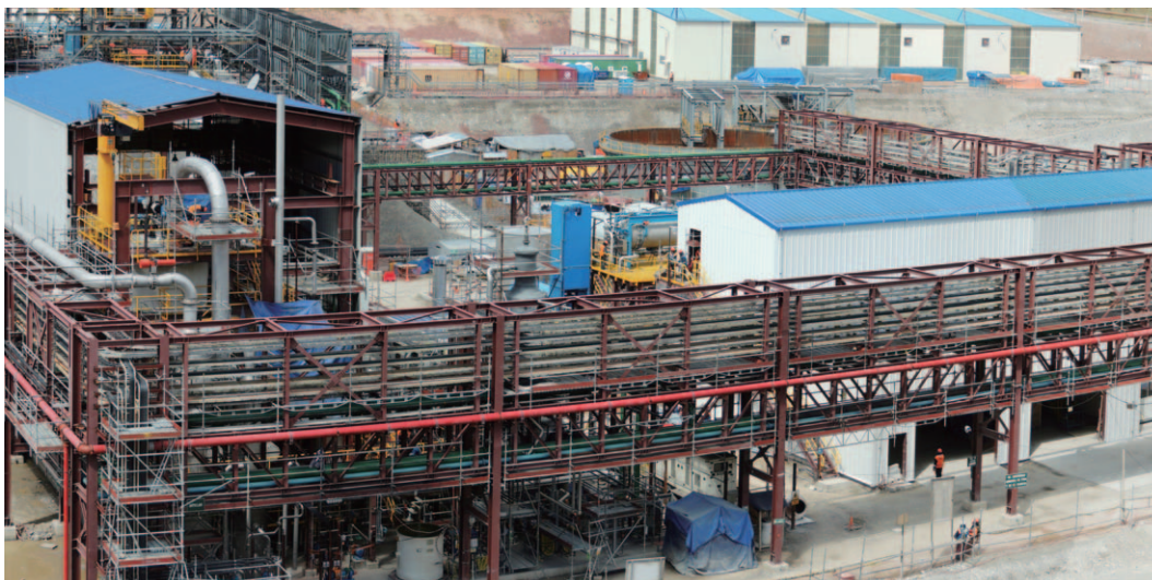
Mo Autoclave Pressure Vessel
