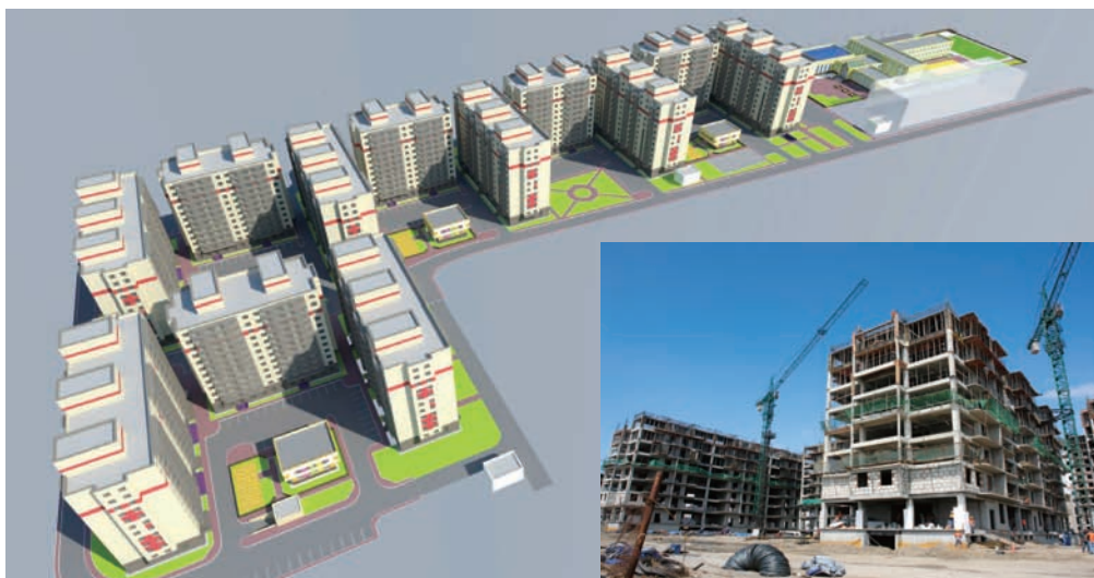
Erin Town in construction
