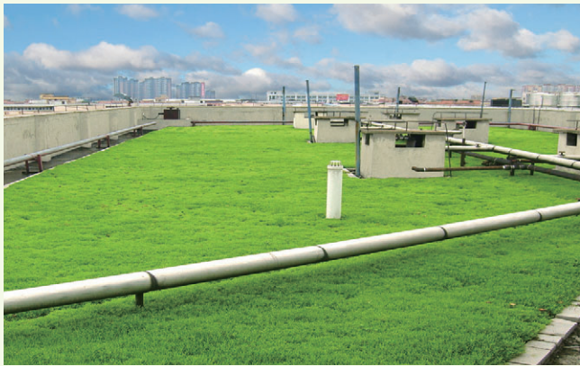
Green roof at ELPs production building
