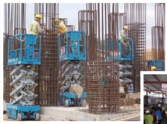
Site Establishment Work
