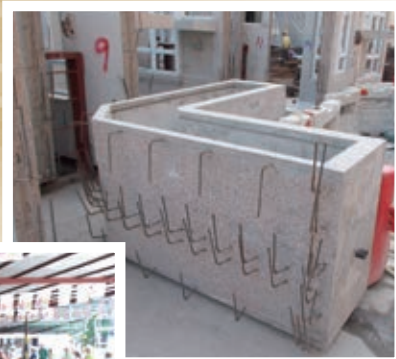
Standardized Precast Work
