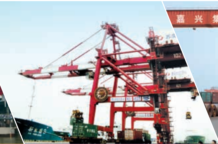
JIANGYIN SUNAN CONTAINER TERMINAL 江陰蘇南集裝箱碼頭
