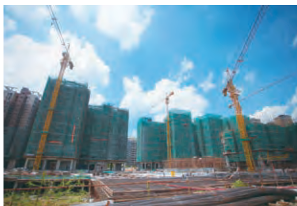
Botanica Phase 3 – superstructure works in progress
