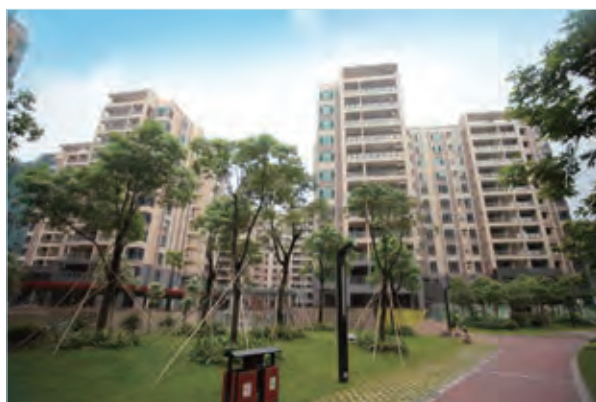
Partial view of apartments under Phase I of Metropolitan Oasis
