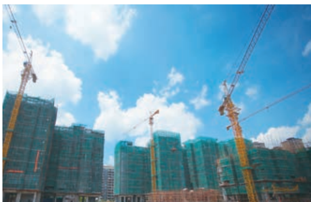
Botanica Phase 3 – superstructure works in progress
