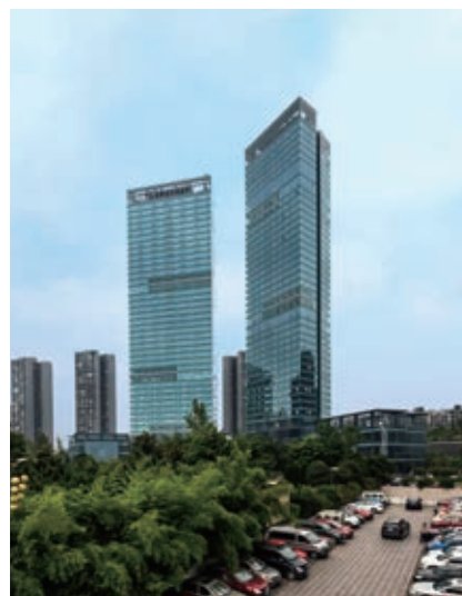
Jinshan Shangye Zhongxin – pending issuance of certificate of comprehensive completion
