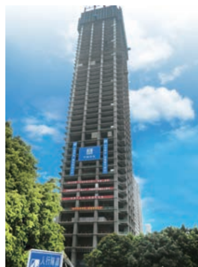
Hon Kwok City Commercial Centre – superstructure works in progress
