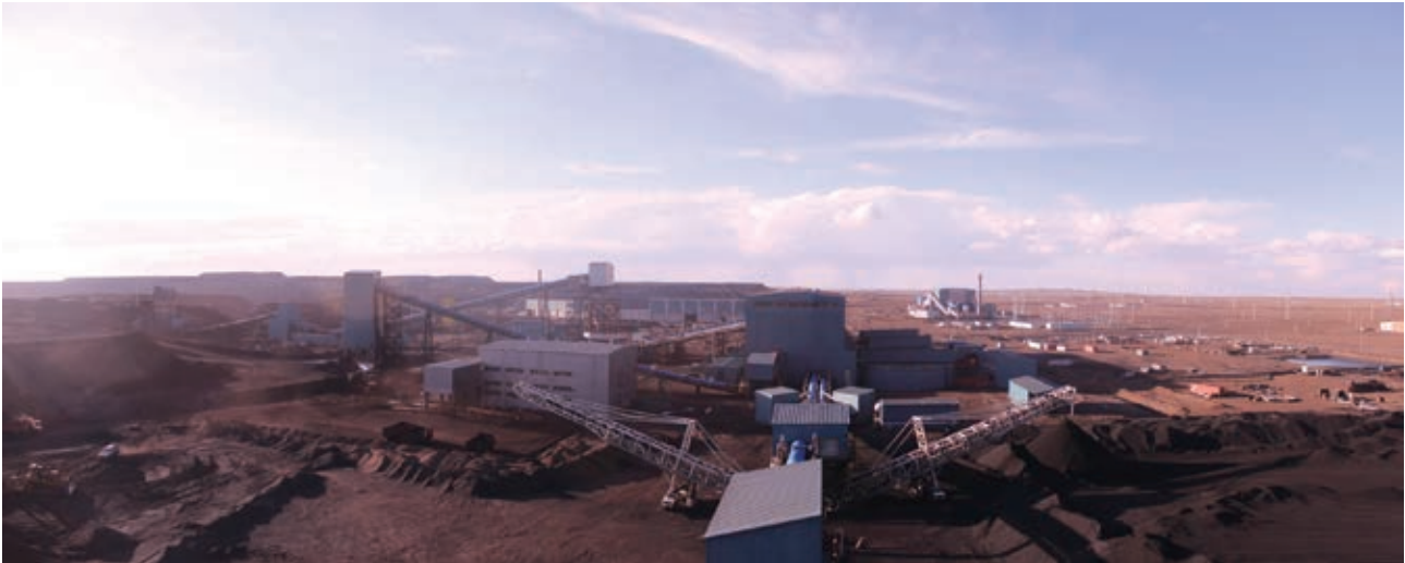
Coal Handling and Processing Plant
