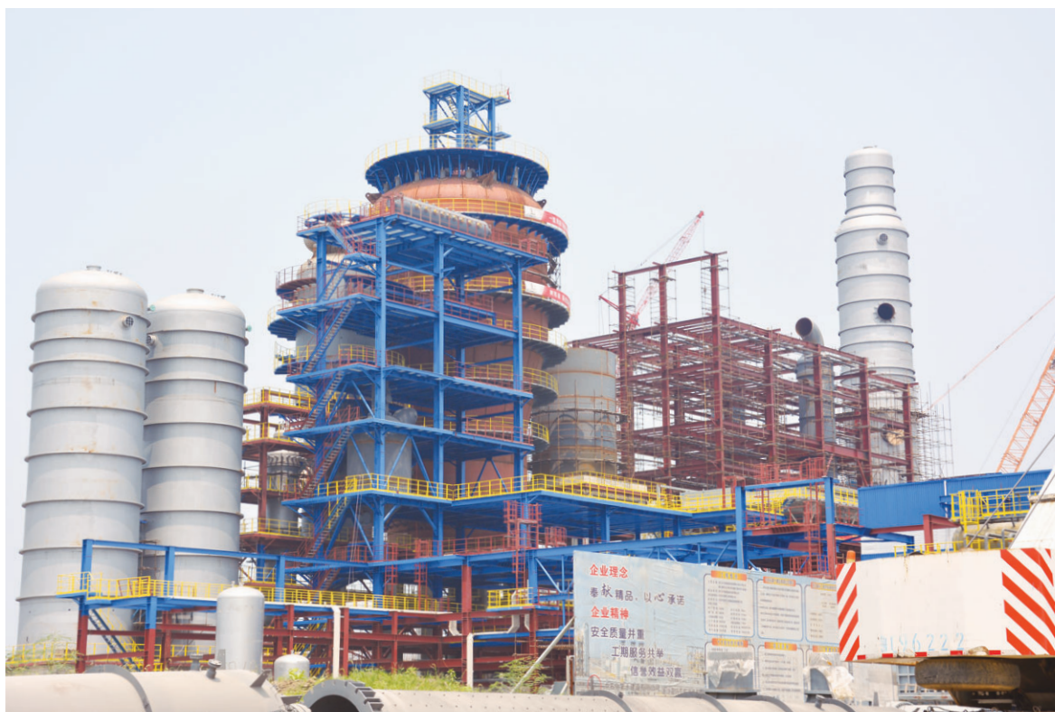
MTO's Reactors & Regenerators (as at Mid-August 2014)
