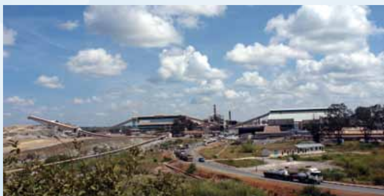
Panorama of the ore processing plant of Chambishi Copper Mine
