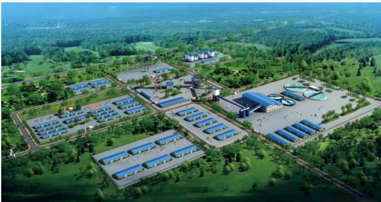
Bird's-eye view of mining and processing engineering of Chambishi Southeast Mine
