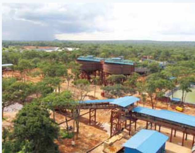
Panorama of 20,000-tonne Mabende Leaching Project when completed
