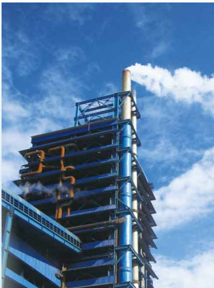
ISA furnace of copper smelting company
