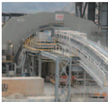
SAG Mill & Conveyor
