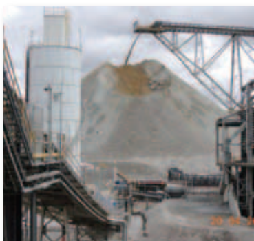
Conveyor & Lime Silo
