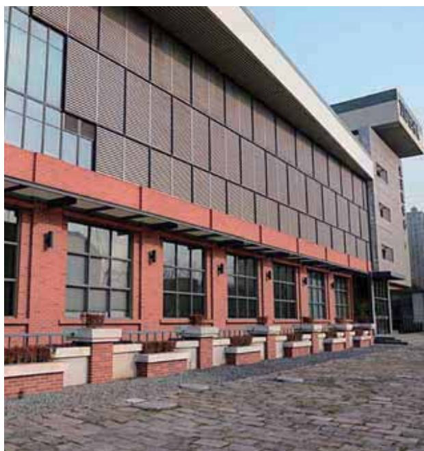
Cloud Computing Data Centre in Baoshan, Shanghai
