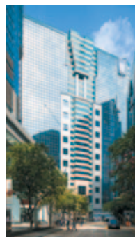
LEE GARDENS TWO/CAROLINE CENTRE 28 Yun Ping Road, Causeway Bay
