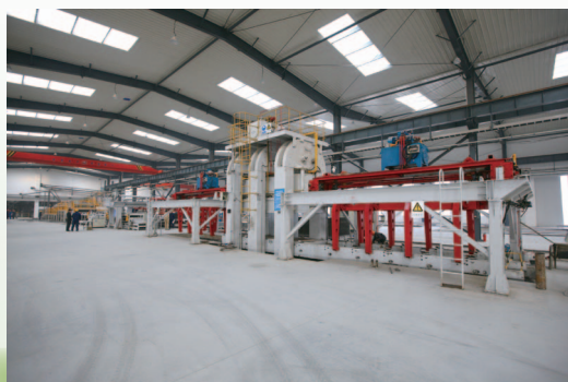
Green Building Material Projects in Bozhou and Wuhu Commenced Operations Successively
