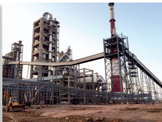
Residual heat power generation project in India under construction
