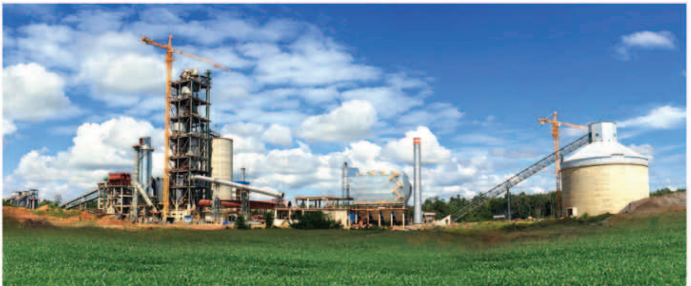
General view of the production line in Kalimantan Conch
