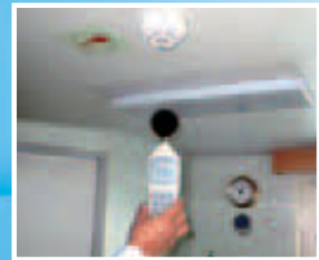
⊕ After rectification: noise is below the national standard of 60db
